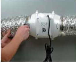
Attach the ducts with clamps.
