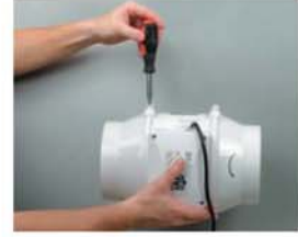
Secure latches by screws.
