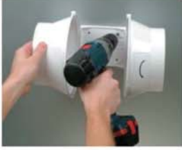
Fix the fan mounting plate on the flat surface.
